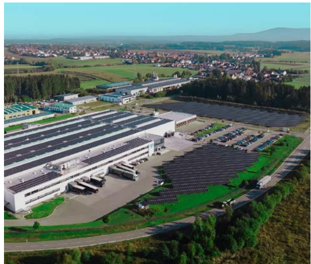
Photovoltaikanlage in Trossingen
