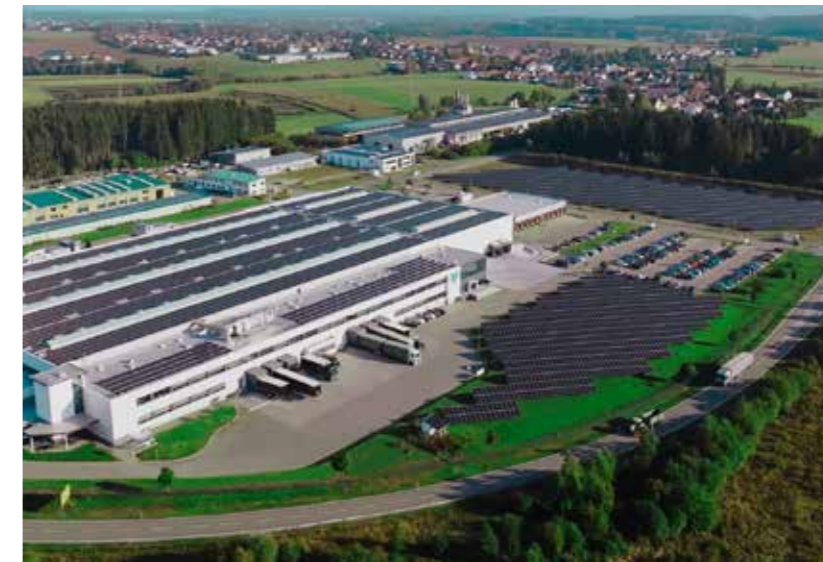
Photovoltaikanlage in Trossingen
